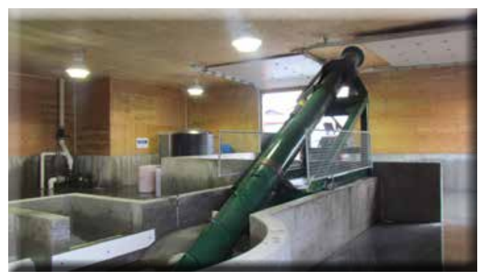
One Shot Sand System used in vortex pit design.
